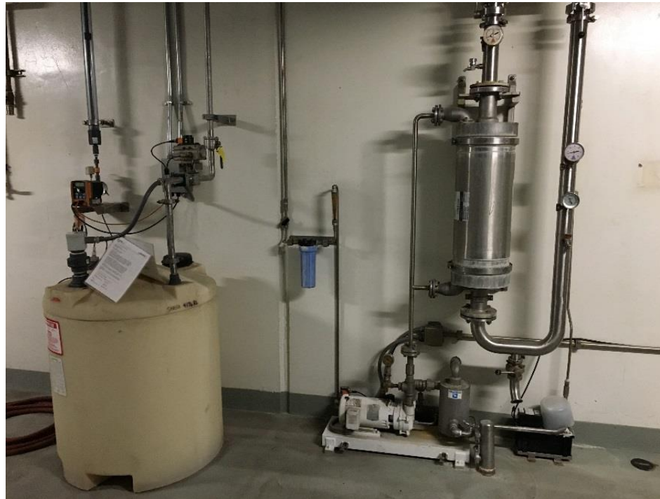
Phosphoric Acid Dosing and Oxygen Reduction
